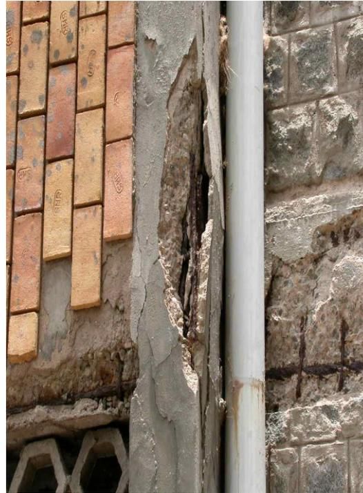
Concrete block with severe cracking caused by DEF and testing of cores by thin section microscopy and residual expansion measurements
